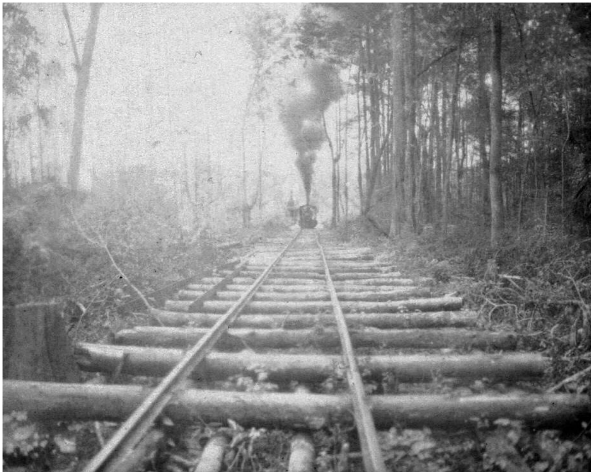
In a lot of places, logs were placed crosswise and the track laid on them as the peat bog didn't provide a firm bed for the track. 2-6-2 #55 shown here. International Paper Photo
